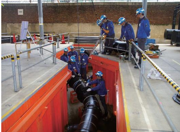
Jointing Large-Diameter Distribution Pipes
