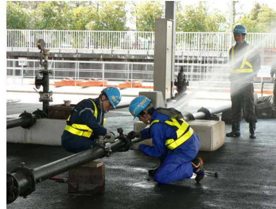
Emergency Remedy of Leakage
